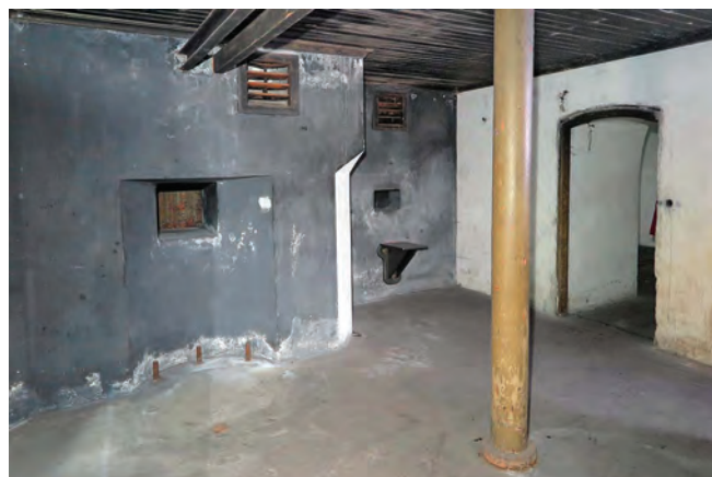
The well-preserved interior of the caponier, showing firing positions. The wooden ceiling was added to reduce the likelihood of injuries caused by splinters of concrete injuring occupants in the event of a direct hit
